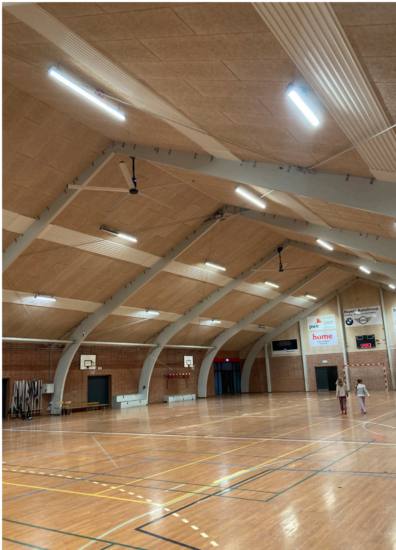
HVLS Ventilatorer, Lyshøjhallen
